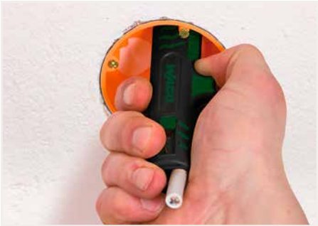
Stripping a cable sheath.
