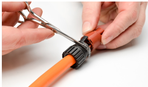
Step 14 - Trim shield as shown
